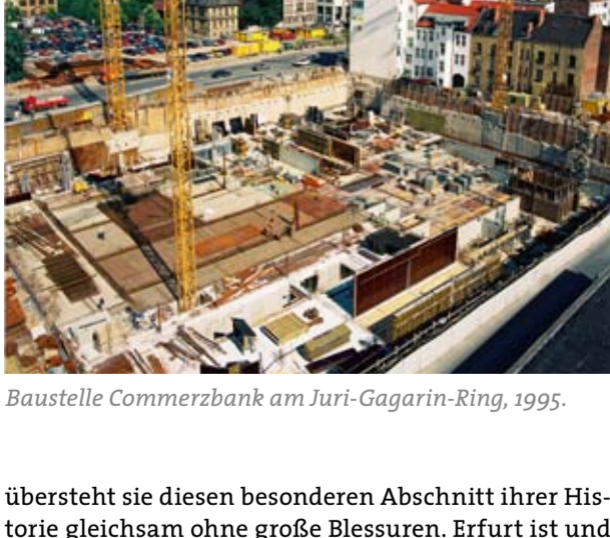
Baustelle Commerzbank am Juri-Gagarin-Ring, 1995.
