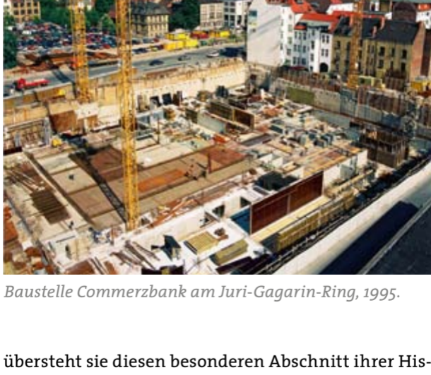
Baustelle Commerzbank am Juri-Gagarin-Ring, 1995.
